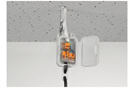
Pendant light connection in a suspended ceiling
